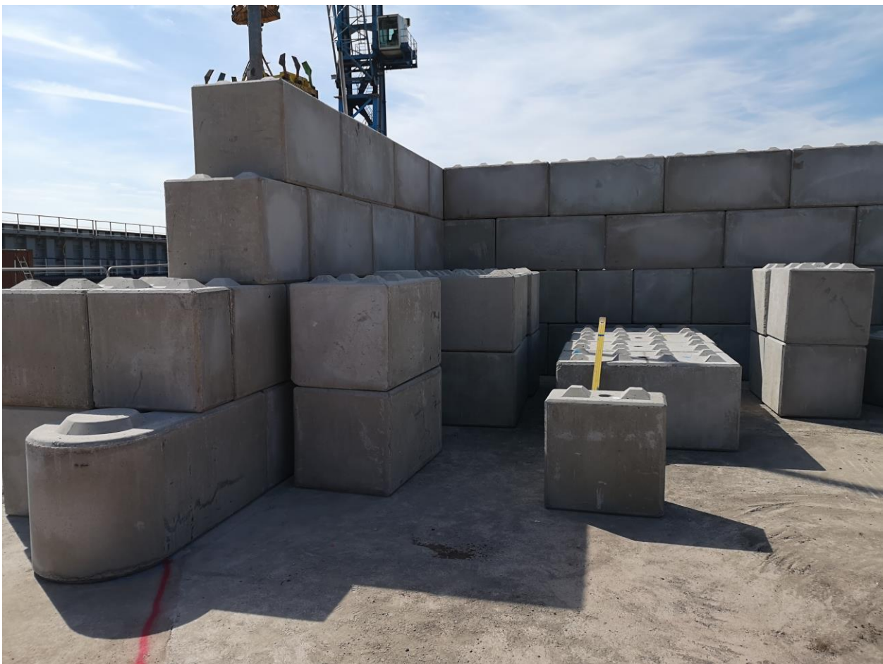
Figure 3: Legato blocks during assembly
